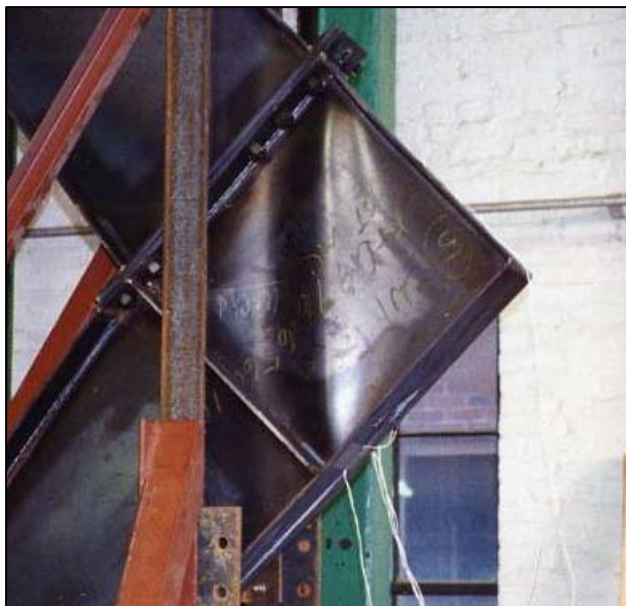
Figure 4.7 Buckling in knee web of frame 3
