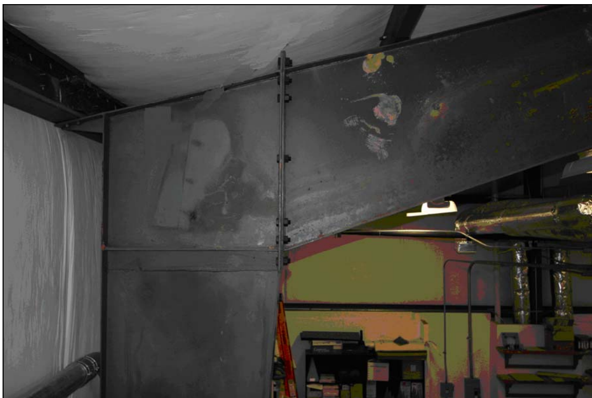
Figure 1.2 A commonly used design for a square knee joint (from figure 1.1)
