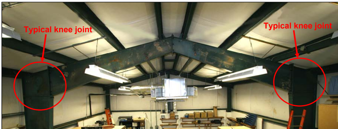
Figure 1.1 A typical frame showing a commonly used square knee joint design
